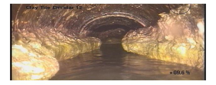
Fats, oils, and grease can also cause interference at the wastewater treatment facility (WWTF). The FOG can negatively impact operations resulting in improper treatment of pollutants. These pollutants that are otherwise removed by the treatment process could be discharged to the waters of Ohio.
