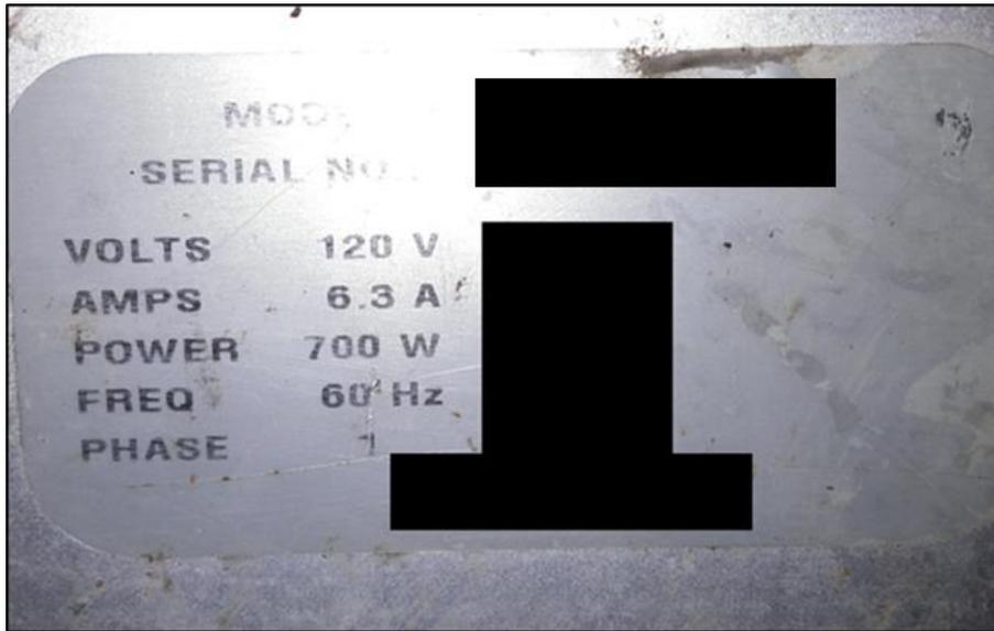
Figure 1. Label on current UV module device (McFarland WWTP, 2021).
